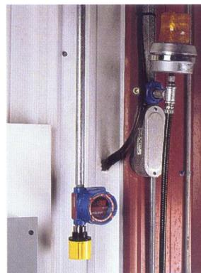
*Intellisense® heads can be powered by a local supply for stand alone, single gas monitoring and alarm .*
