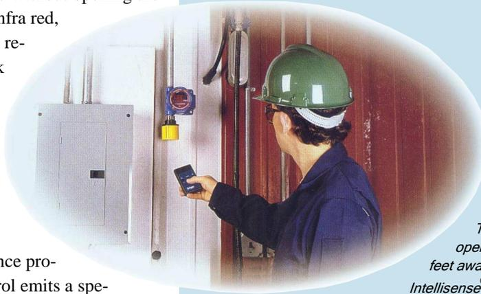
The remote control is operational from up to 12 feet away from the Intellisense® sensor.
