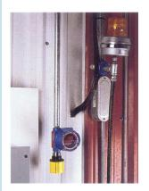
Intellisense<sup>®</sup> heads can be powered by a local supply for stand alone, single gas monitoring and alarm.
